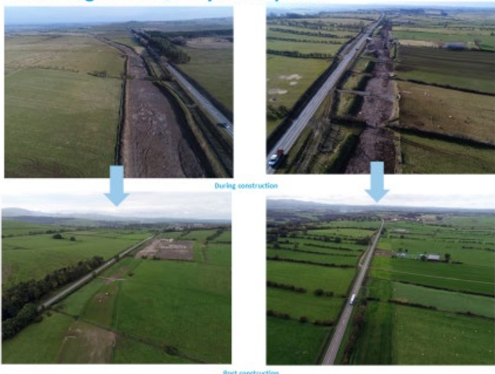
Williamsgate to Quarry Hill Pipeline
