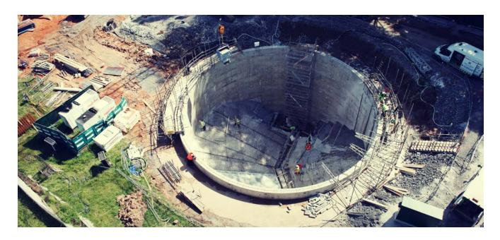
**Pictured:** Construction of a storm tank as part of a £5 million sewer improvement scheme in St Helens. Underground tanks such as this help to store huge amounts of water during heavy rainfall, preventing flooding.
