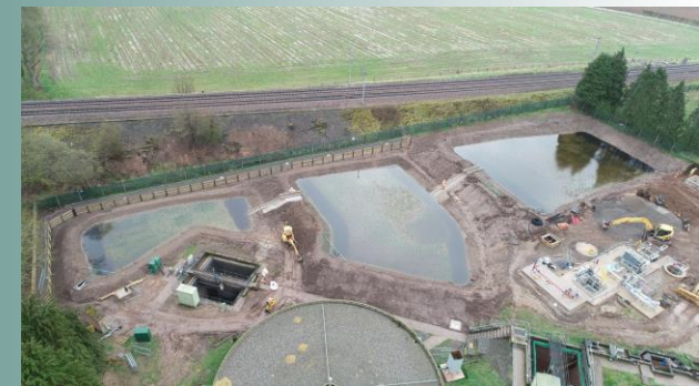
Southwaite wetlands under construction
